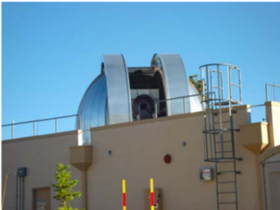
Figure 72: OCTL telescope will be modified with an optical flat to support links in the presence of more windy conditions.
